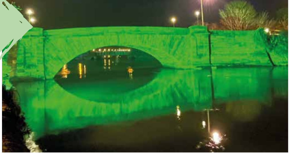
Devonshire Bridge, Dungarvan, Waterford.
